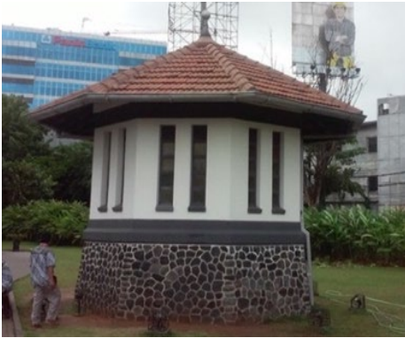
Figure 4. The Well Pump House
